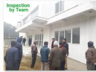
Construction team visit at CKNEH-Bahadurgunj.
